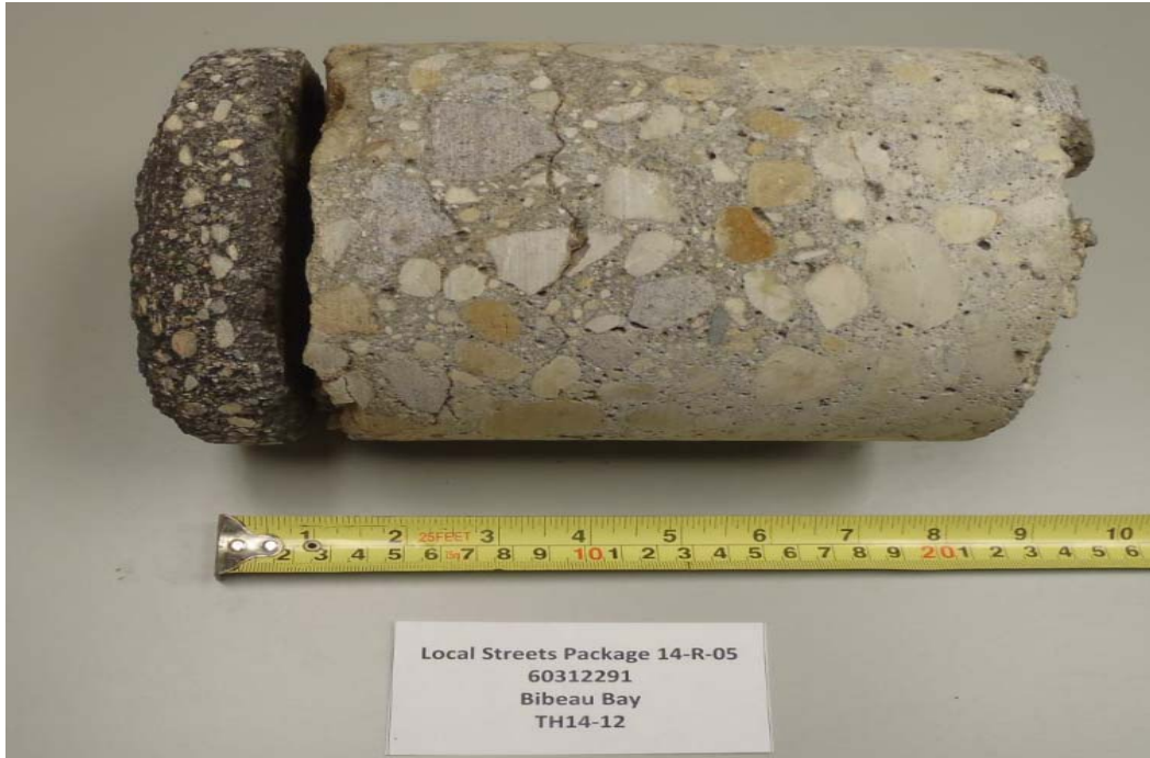
Photograph 7. Bibeau Bay – TH14-12
