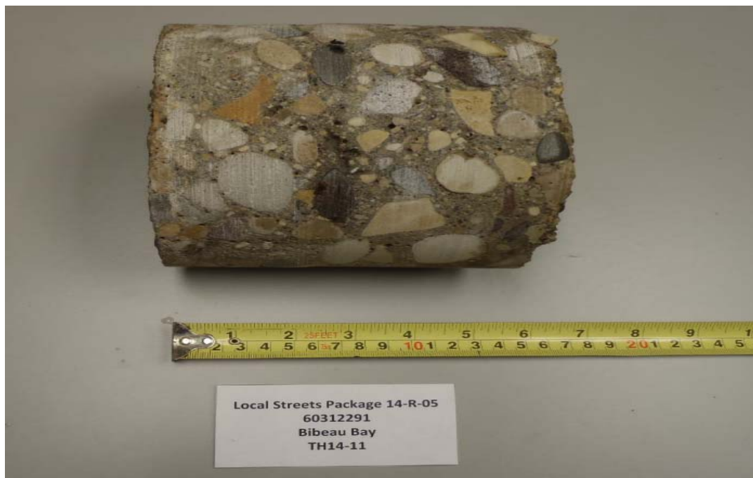
Photograph 6. Bibeau Bay – TH14-11
